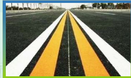
Thermo Plastic Paint with application
