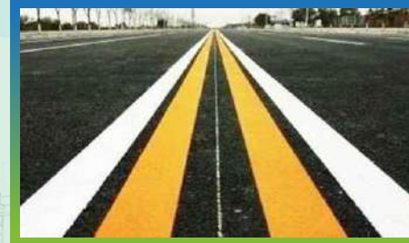
Thermo Plastic Paint with application
